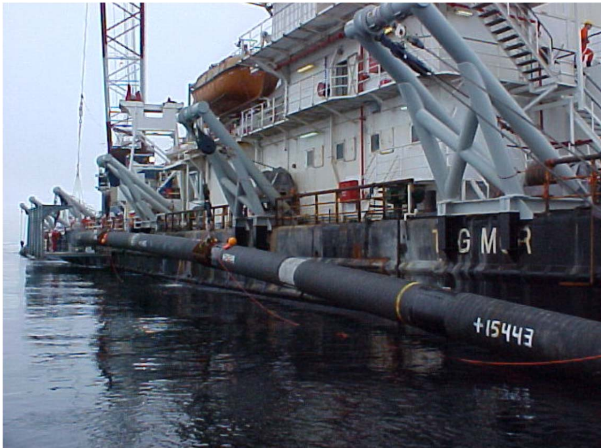
Figure 2.17: Typical Above Water Tie In Operation
