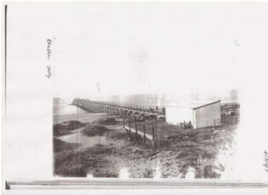
Figure 5-15: Timber Jetty at Onslow
