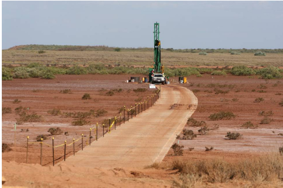
Photo # 13: Using Dura-Base mat to construct a temporary access over intertidal marshland. This prevented vehicles from bogging, which avoided clearing that would otherwise have resulted from repeated track widening and bog recovery works.
