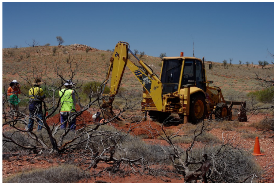
Photo # 4: Typical geotechnical test pit activity.
