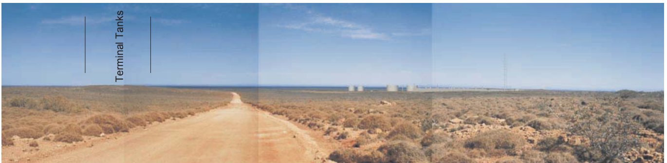
Figure 3.19 – Simulation of LNG Plant at completion of works from Viewpoint 7 – Ridgeline West of Terminal Tanks
