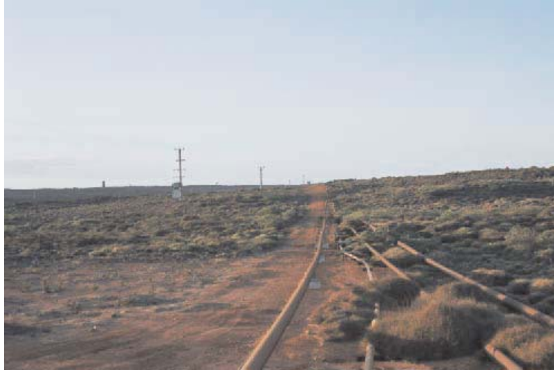
Fig 2.22 Viewing south showing typical pipeline and power easement at junction of north south and east west roads
