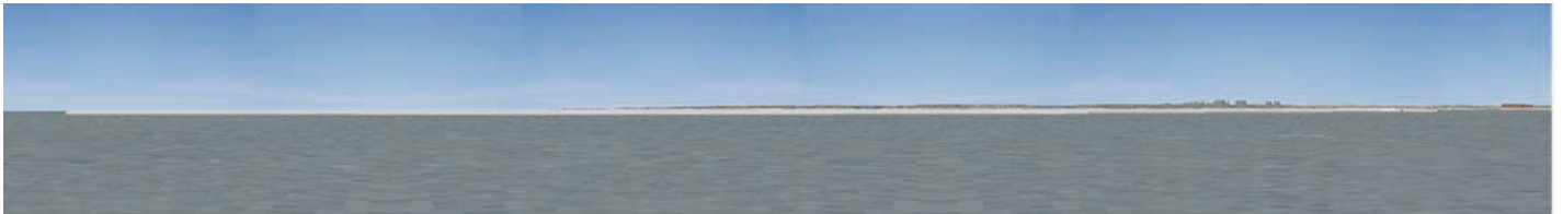
Figure 3.13 – Simulation of LNG Plant at completion of works from Viewpoint 4 – Ocean View at 5km east of LNG Plant. View at left of figure shows extent of Ship Gas Loading facility.
