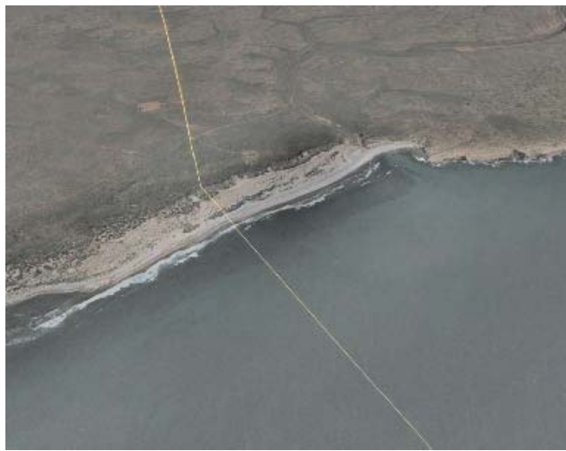
Fig 3.1 Aerial viewing east towards White's Beach showing proposed pipeline corridor and existing road running adjacent to shoreline.
