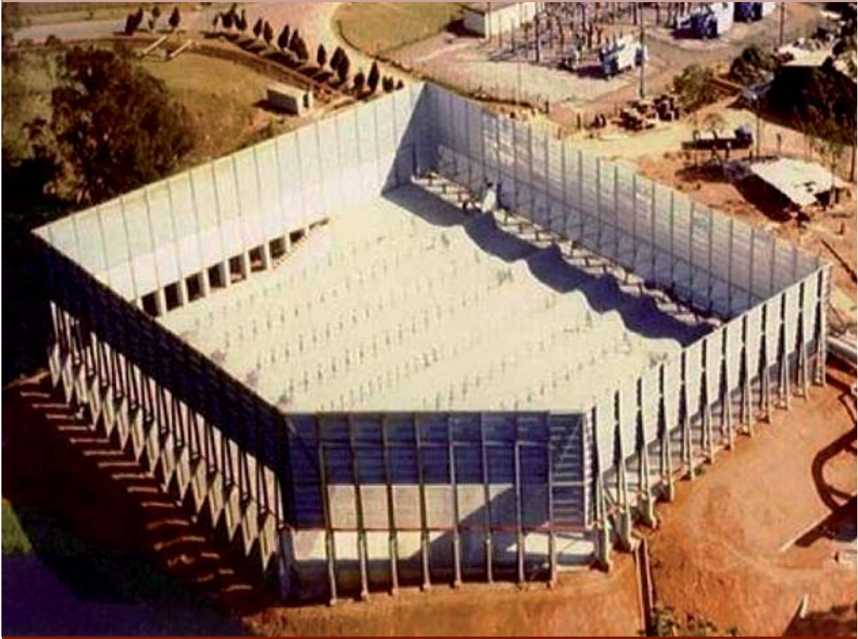
Figure 19: Typical Ground Flare
