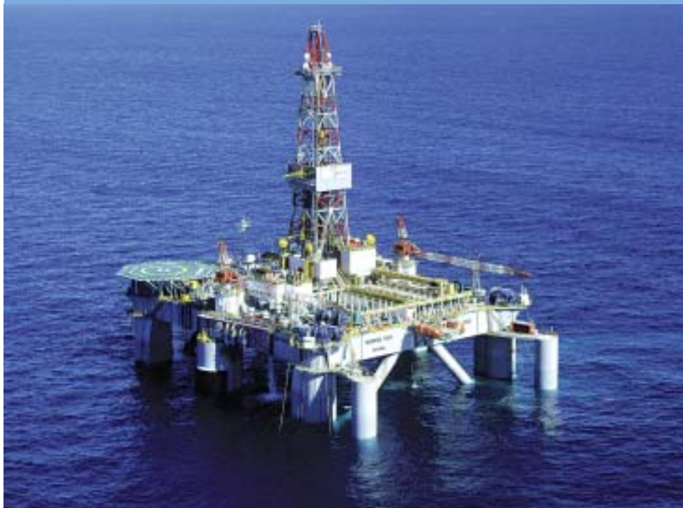
Plate 6-1: Typical Drilling Rig used in North-West Australia
